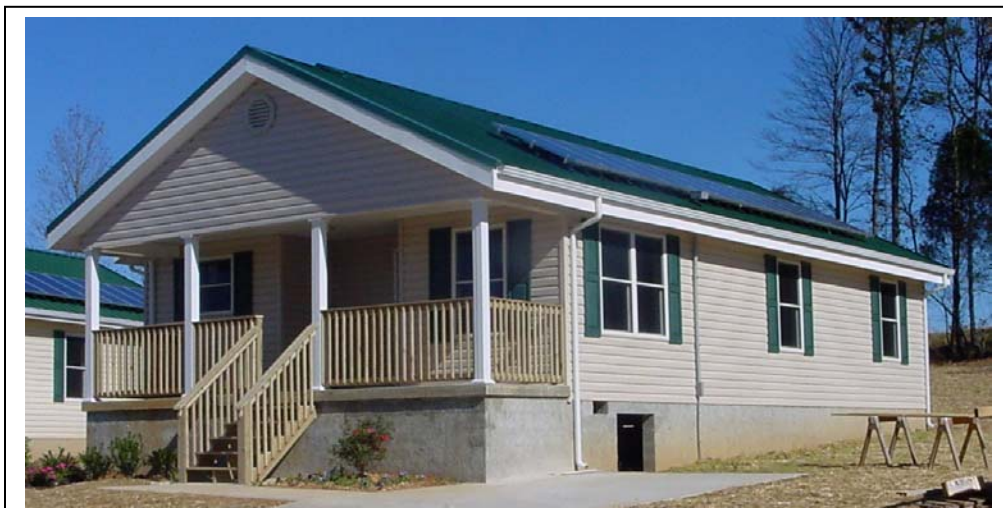
Figure 13 ZEH3 has only 12 solar modules compared to ZEH1 48 and thicker SIP roof and walls.
