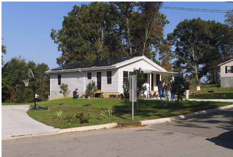
Figure 2 ZEH1 showing the 48 roof mounted solar modules and south facade
