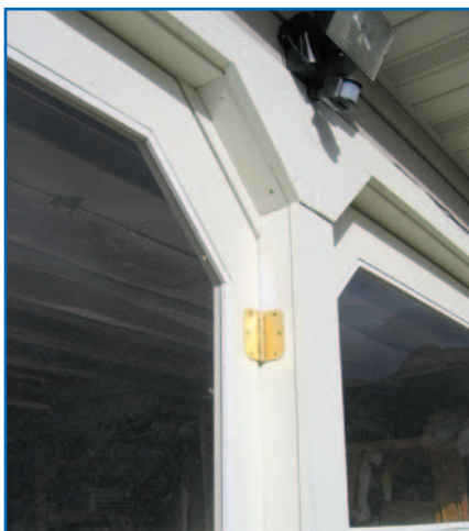
Outside view of the removable center column, trimmed to match the existing frame.
