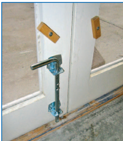
Inside view of the bottom of a door pair, without trim strip installed. Toggles hold summer reflector panels in place.
