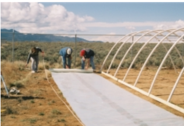
Figure 9. Rolling out the plastic to the appropriate length.
