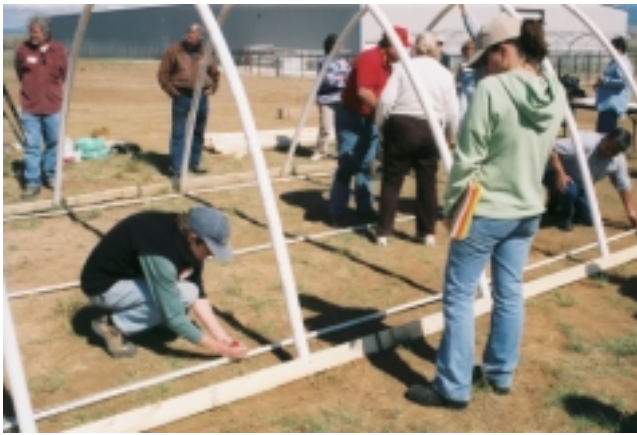
Figure 5. Laying out the tubular 3/4-in. braces.
