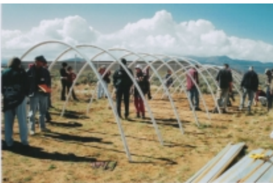
Figure 3. The hoop house structure takes shape.
