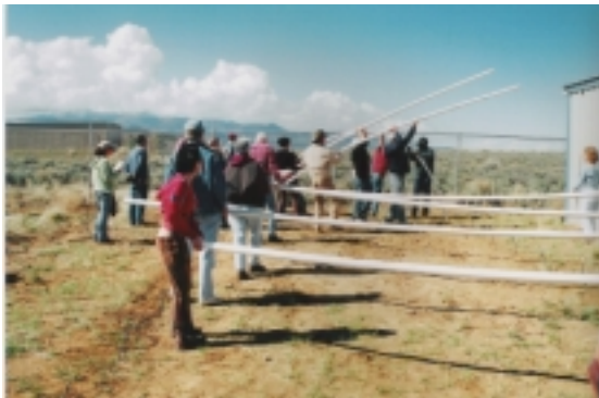
Figure 1. Laying out the 2-in. x 20-ft. PVC pipes that will be used for the frame.
