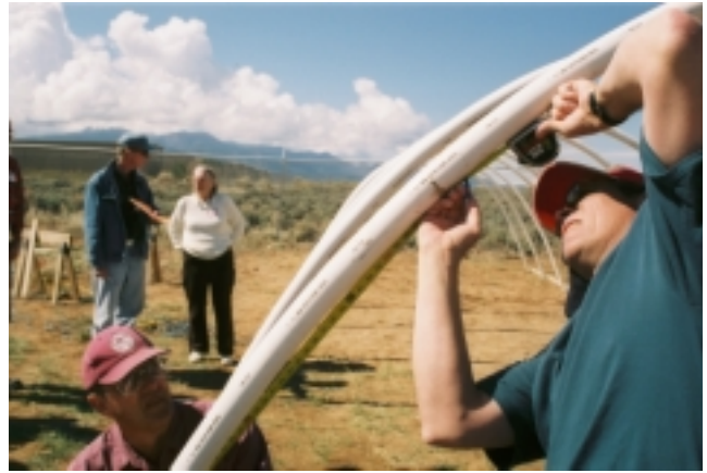
Figure 6. Marking the height where the braces will be attached.
