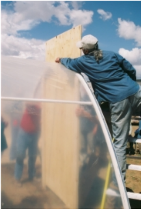
Figure 13. Marking the door to be cut.
