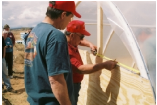
Figure 16. Making a window on the back end wall.
