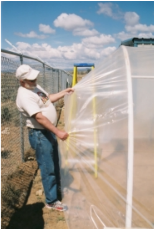
Figure 11. Stretching the plastic over the hoop house structure.
