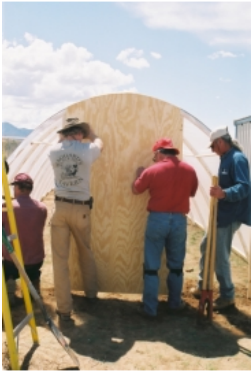
Figure 14. Attaching the front door to the hoop house.
