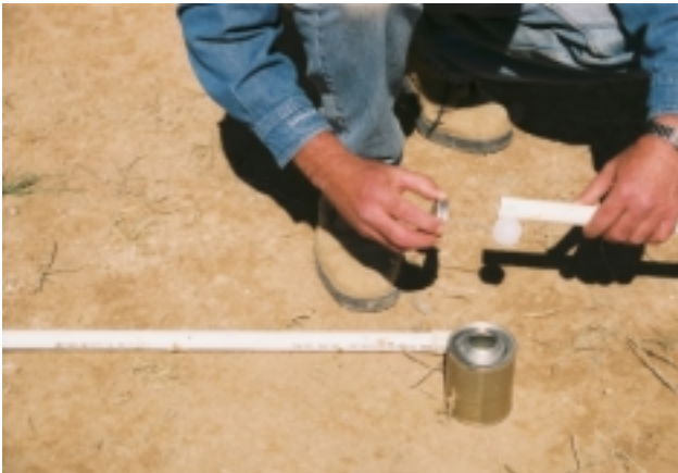
Figure 7. Gluing 3/4-in. pipe together to be used as braces.
