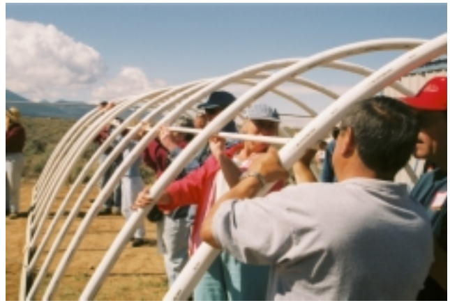
Figure 8. Attaching the 3/4-in. PVC pipe braces to the structure.
