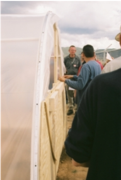
Figure 17. Window completed; hoop house completed.
