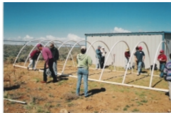
Figure 4. Attaching the baseboards to the bottom of the PVC pipes.
