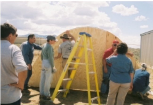
Figure 15. Finishing the front end wall of the hoop house.
