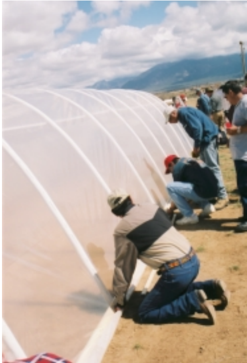
Figure 12. Attaching the plastic cover to the baseboards.
