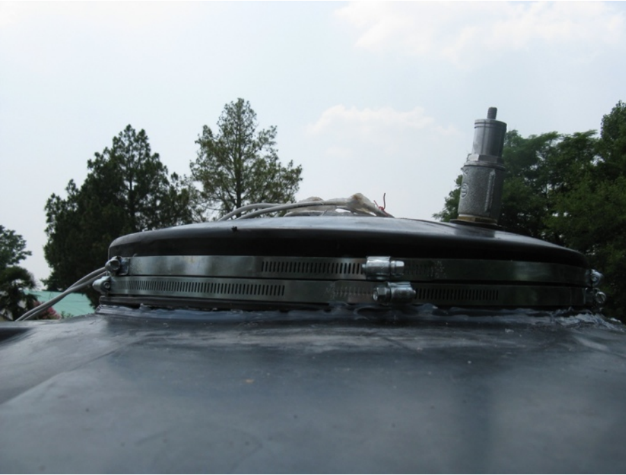
Bulging lid - the rest of the tank is similarly bloated.
