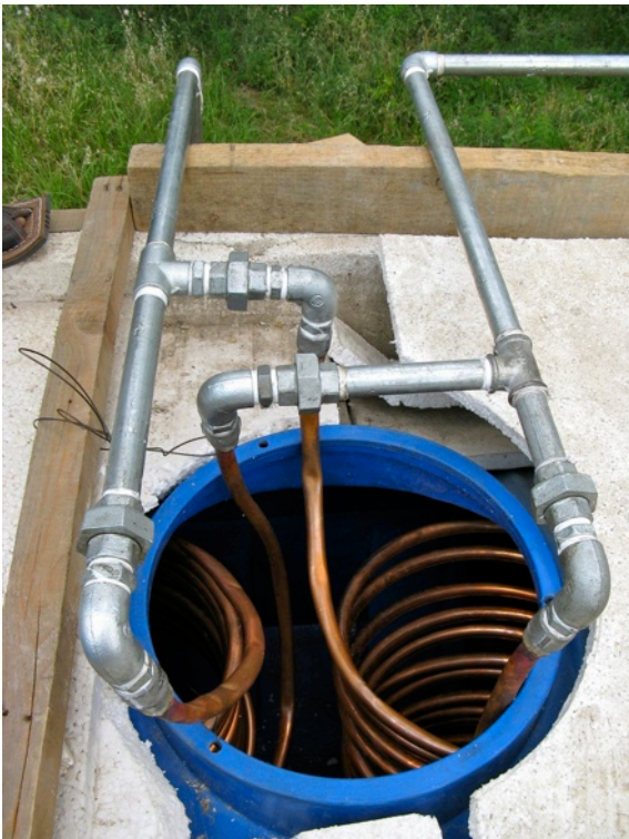
Heat exchanger in place.
