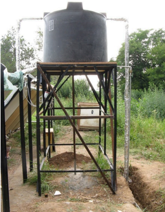
New tank atop reinforced stand.
