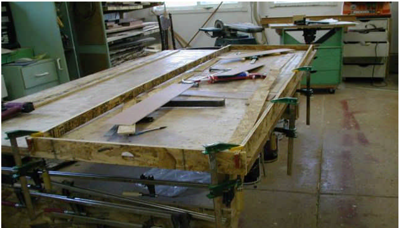
Basic frame set together with construction adhesive clamped to table to keep it square. The hole shown is the central drain.
