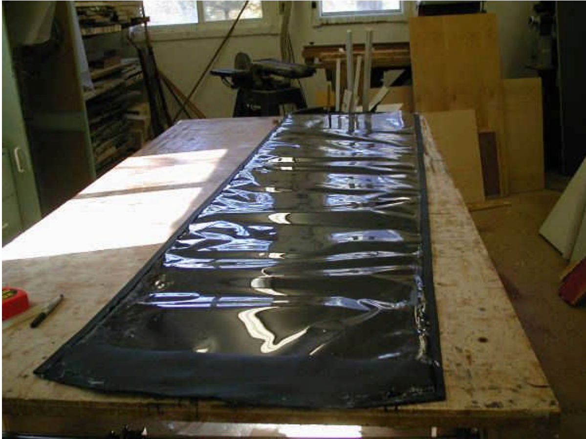
Sides glued down and second standing seam along bottom of funnel done. Top of funnel is still open.
