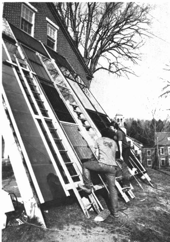
Roof Glazing Systems Test
