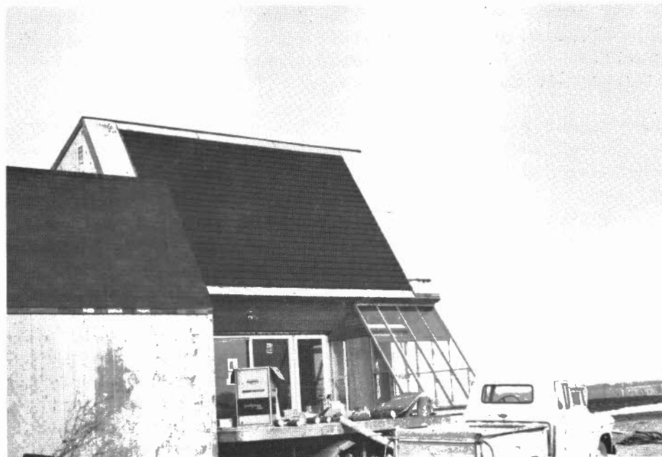
Active Solar Collector Construction
