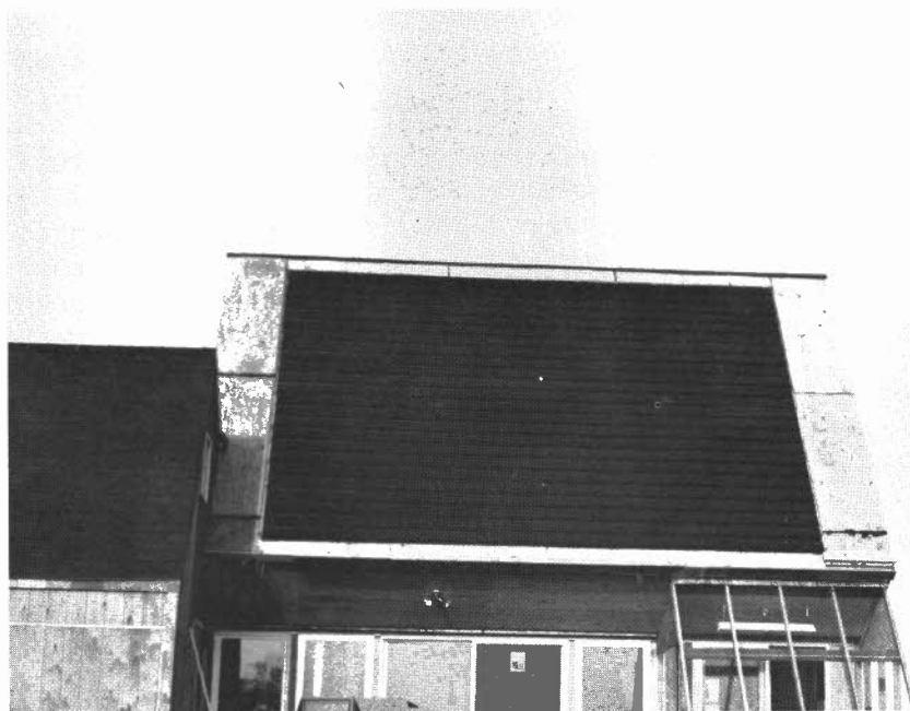
Painted Absorber Plate
