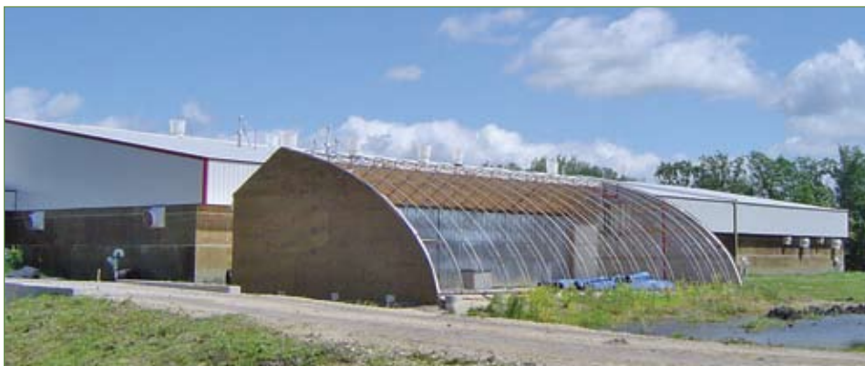
An experimental hog finishing barn and partially constructed solar greenhouse on the grounds of the University of Manitoba's Glenlea Research Station. A new study is set to test the feasibility of supplementary heating for solar greenhouses using warm, biofiltered air from the hog barn.
