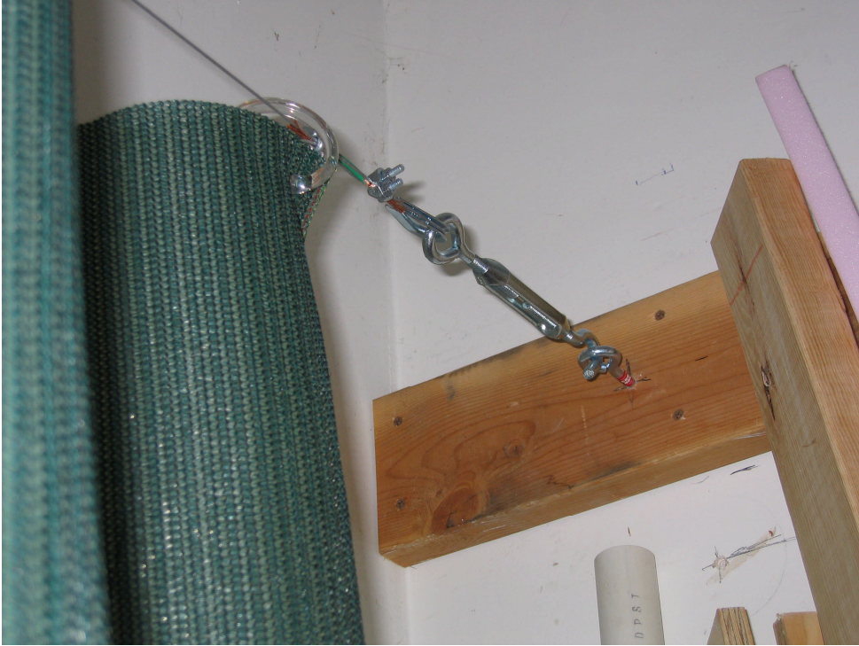
Shade Cloth, shade cloth support wire and turnbuckle. One of the shower curtain sliders is also visible near the top of the picture.
