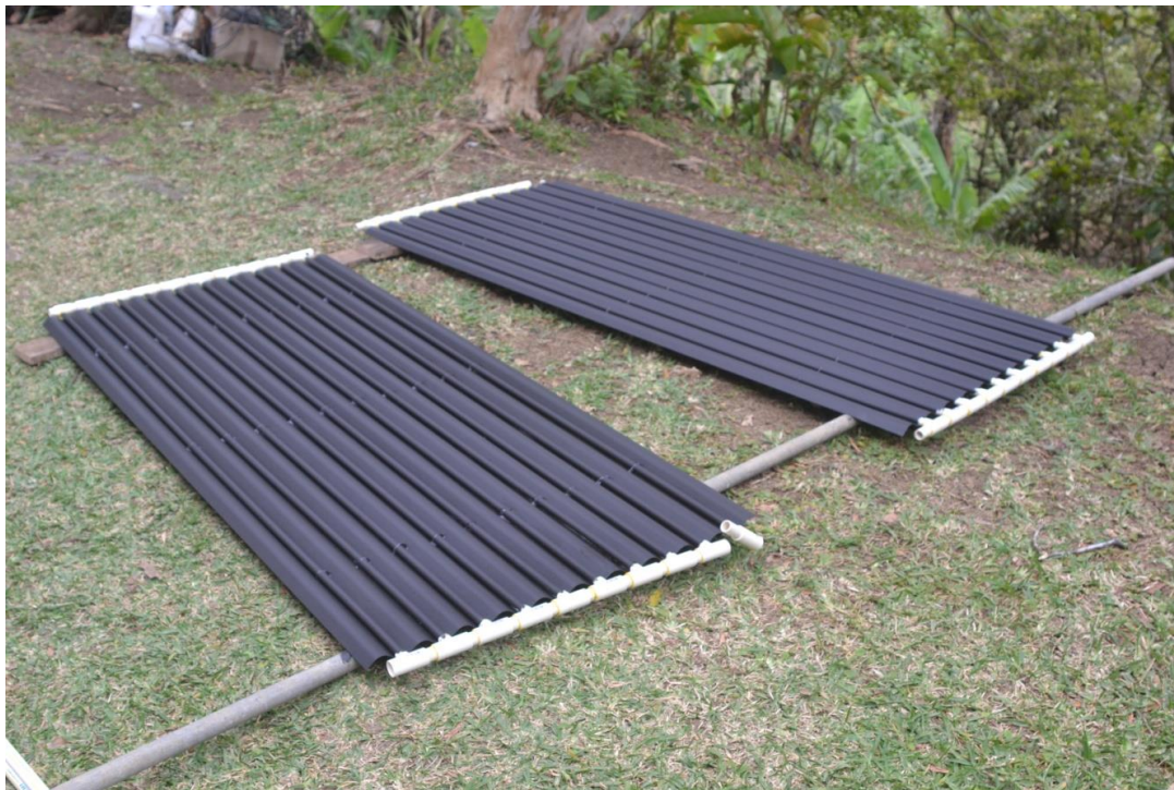
Painted and ready for the roof
