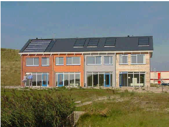
Figure 1: The 4 test houses at ECN, labelled 'A' (at the left) to 'D' (at the right). PV is integrated in the roof of the leftmost house (the 'A-house').
