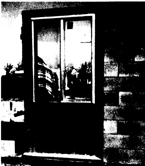
Figure 15.—Prefabricated wood frame window panel with exterior finish of rough-sawn plywood.
