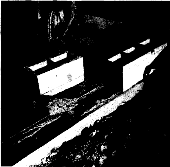
Figure B.-Lay the first course of blocks in rich mortar on the slab floor or footing.
