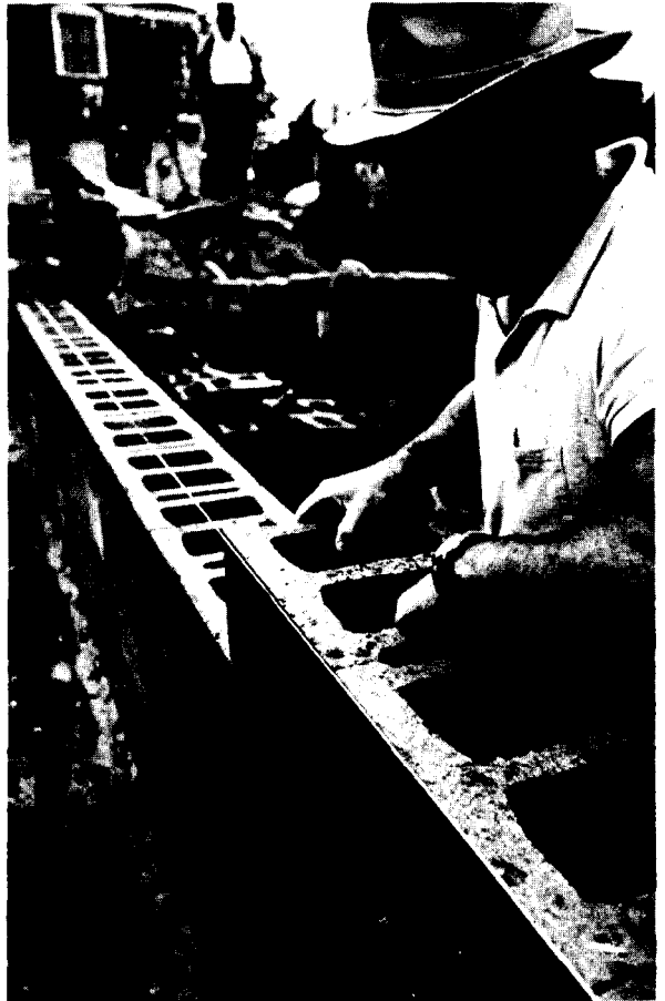
Figure 8.-Mason's line held between corners with wooden hooks. Lay wall without mortar to line.
