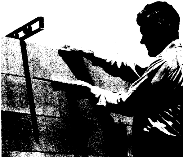
Figure 9.—Insert metal shims between blocks if necessary to level or plumb the wall.
