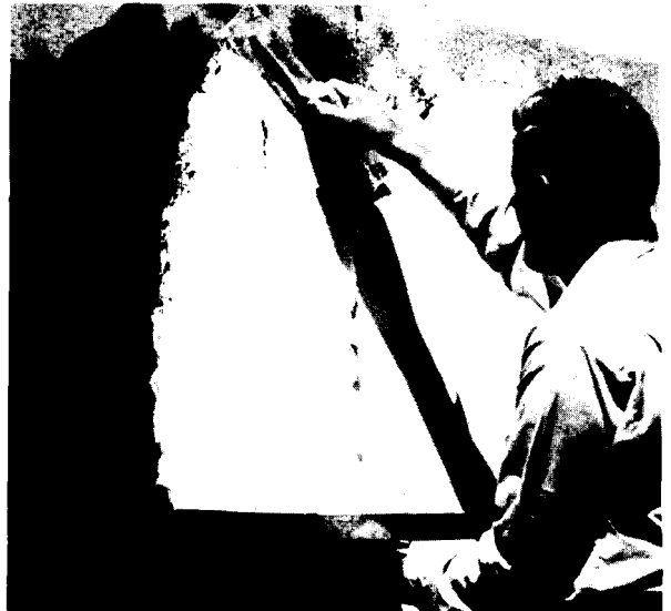
Figure 23.—Work the bonding mix from a hawk onto the wall with a plasterer's trowel. Note the specially made hawk with turned-up edges on three sides to prevent spilling the relatively thin mix.
