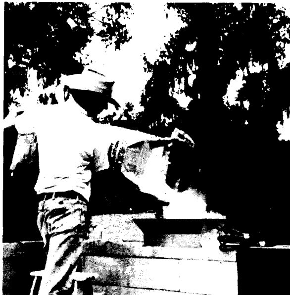
Figure 19.—Filling cores of concrete block wall with pellet insulation. Rectangular metal funnel made to fit the width of the wall reduces the filling time and avoids spillage.
