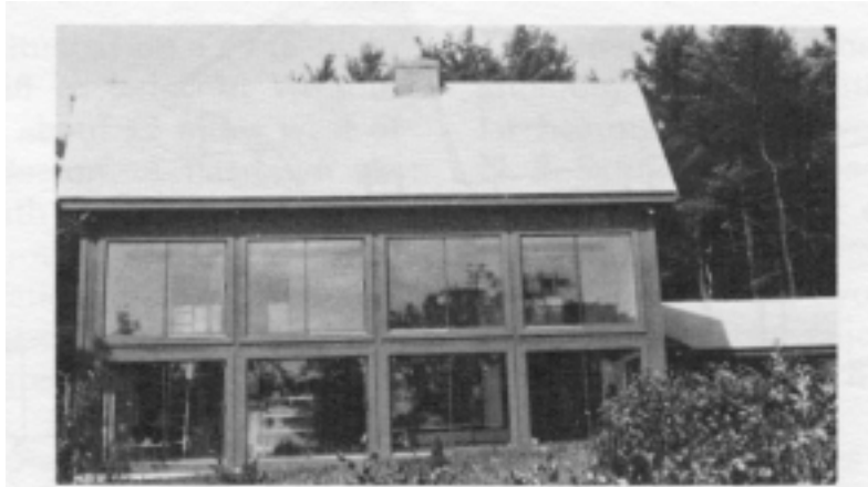
South face of Cliff House sunspace, showing the eight double-glazed windows.
