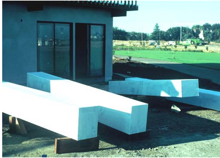
Low water wall tanks primed and ready to paint and install
