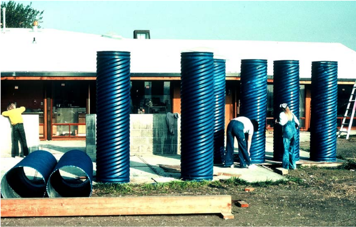
Culverts installation for a day care center
