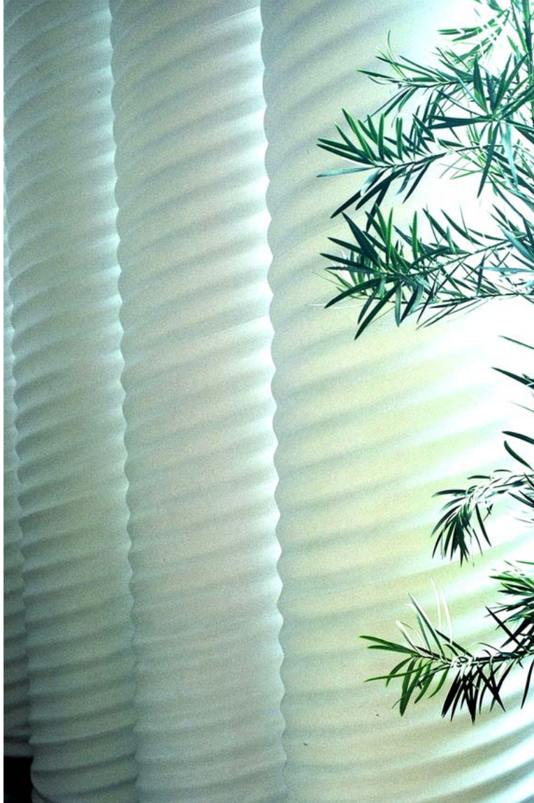
Culvert wall at Living Systems Office, Winters
