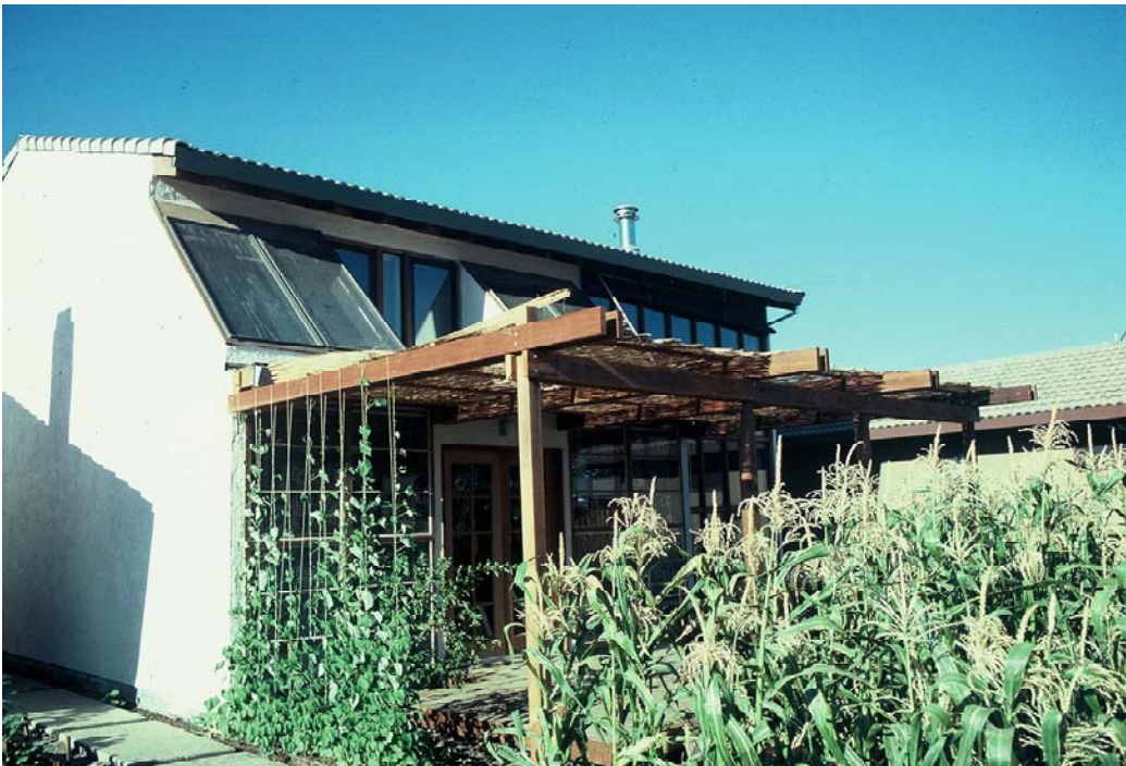
Culvert wall house in Davis, 100% natural cooling, 70+% natural heating, integral solar water heater.
