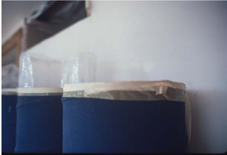
Plastic lined sheet metal tube water wall, BC
