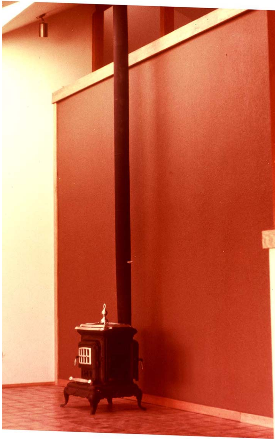
Big water wall tank behind stove, Village Homes
