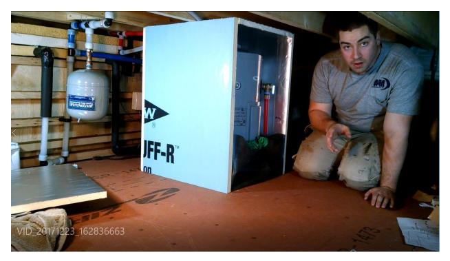
Electric booster tank inside an insulation box.
