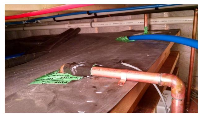
Pipes entering the tank through the lid with gasketed seals. Note the temperature sensor is taped to the copper pipe.
