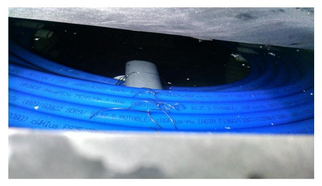
Filling the tank with water above the heat exchanger.
