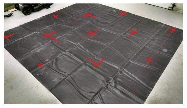
Chalk lines snapped out on EPDM prior to installation.
