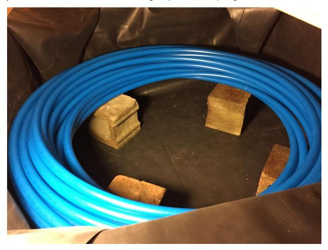
Coil of PEX tubing inside tank, 300 feet, one-inch nominal.
