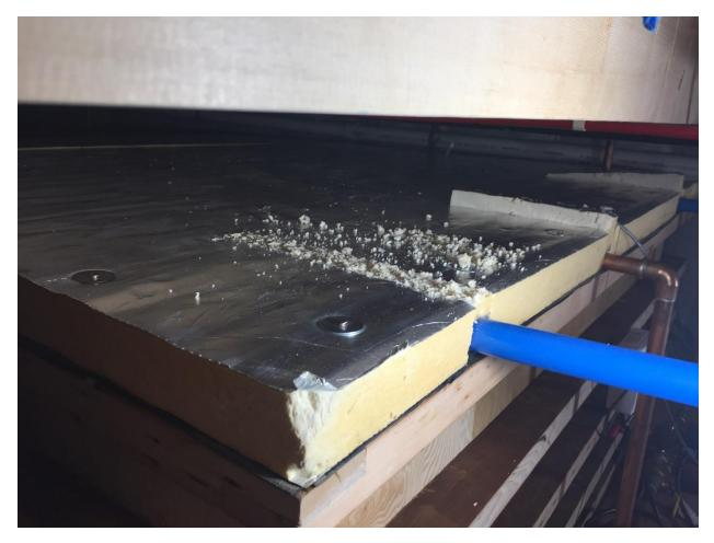
First layer of foam is screwed in place, and cut to fit around pipes.
