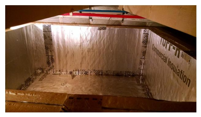
Foam insulation in place on walls.
