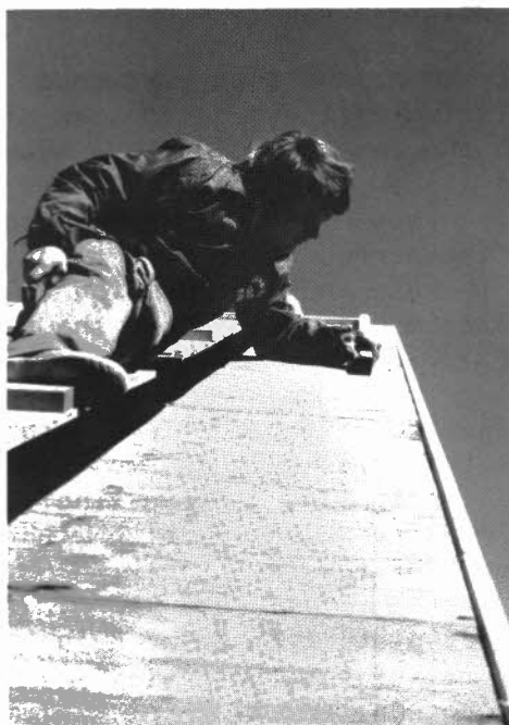
Tacking the Perimeter Blocking
