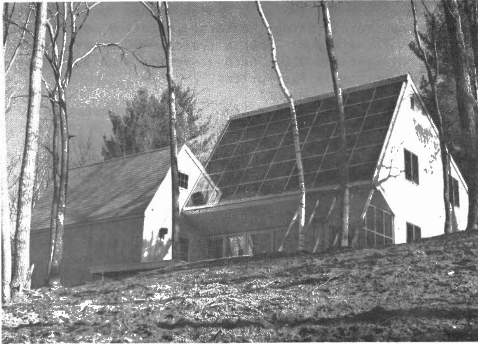
A Site Built Active Solar Collector Installation
