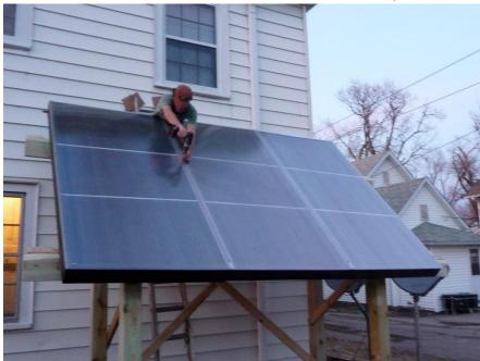
Aluminum trim on collectors and use of off-the shelf "joiners" for the glazing.
