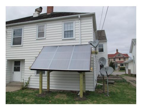
This ground-mounted drainback system follows the design and build instructions from Gary's site with a few minor exceptions. The system provides an undetermined percentage of the domestic hot water for a seven-unit apartment building in Southeastern Iowa (41 degrees latitude).
