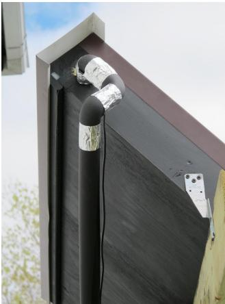
I soldered the ¼" manifolds parallel to the frame of the collector. To get the needed slope for drainback, the ground mounted rack is sloped ¼" per foot.
