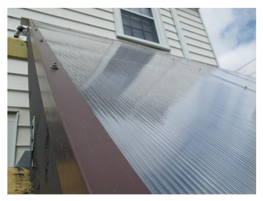
The sides and top of the polycarb sheets are screwed directly into the frames (using screws with rubber washers also sold with the polycarb sheets). Then I bent some aluminum flashing to cover the entire top of the collector and sides halfway down. This gives the collector a more finished look and will protect the wooden collector frame (I also painted this with black deck stain).
