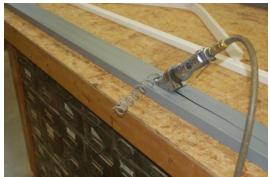
The lid for my tank was not big enough to solder everything together outside of the tank first. So I had to place the bottom manifold in first, then one coil at a time, and finally the top manifold
