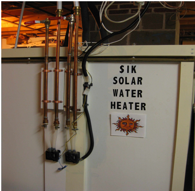
Illustration 6: Note addition of second pump and u-tube to run the third panel
