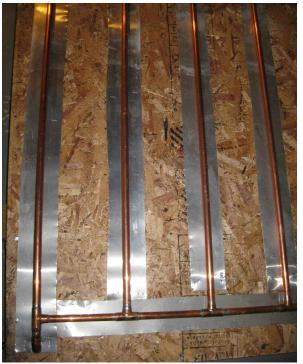
Illustration 4: Three inch strips of aluminum under the copper grid. The strips were painted to avoid galvanic corrosion.
