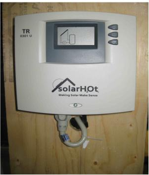
*Illustration 2: Steca 0301 U Solar Controller turns on the pump on and off.*
