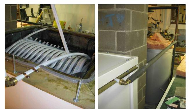
Illustration 16: Heat exchanger in tank. Inlet pipe is foreground.
