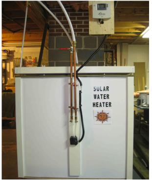
*Illustration 23: The tank and controls. Note the feed and return lines to the tank.*
