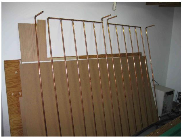
Illustration 3: Copper grids soldered and awaiting placement on the collector panels
