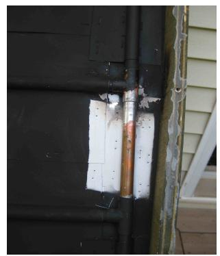
*Illustration 22: The leak site after soldering. It held!*
