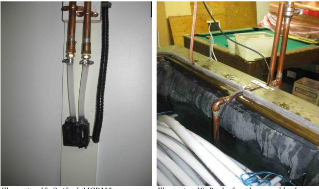
*Illustration 18: Swiftech MCP355 pump uses only 18 watts and is quiet.*
