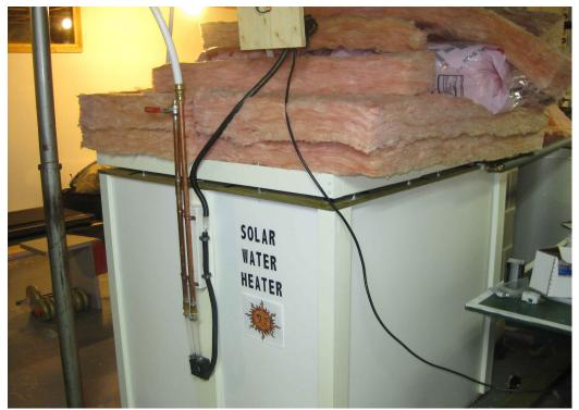
Illustration 6: I decided to store the unused fiberglass batts on the tank....this should increase the R-value of the lid!
