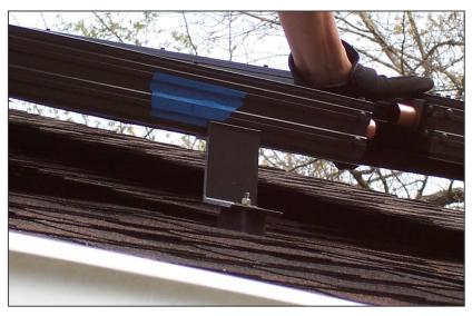
If I had it to do all over again, I wound still use the Quick Mount PVs, but I would set them in a 3 x 3 grid, run U Channel across the QMPVs in 3 horizontal runs, and then mount the collectors to the U Channel "rails" using the AE-RM brackets. In hindsight, this would have made setting the proper drainback pitch as well as aligning the couplings much easier – though with careful planning, measuring and execution, the way we did it was not that difficult.
