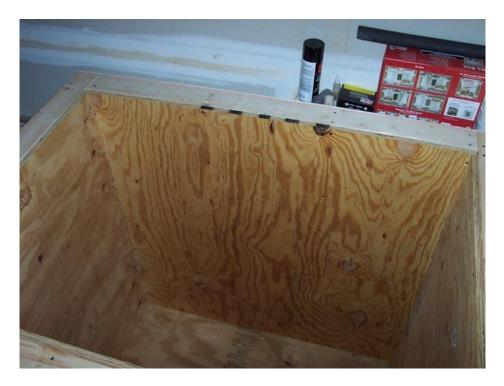
Above is the finished carpentry on the tank. The bottom and side walls are  $\frac{3}{4}$ " underlayment plywood. There is a 5mm luaun plywood cover on the outside to dress it up a bit.
