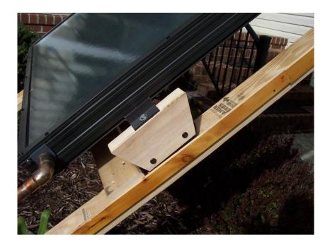
Enlisting the aid of 2 of my ham radio friends, this made rolling the collectors right up onto the roof a relatively simple task. Fortunately, the Quick Mount PV mounts installed by the roofers months before were near-perfectly positioned for the collector mounts to drop right in place. The mounts were placed so that the collectors orient with approximately 3/16" per foot pitch for correct drainback.
