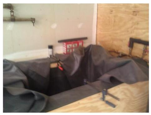
Unfortunately, I did not take any pictures of installing the polyisocyanurate board in the tank, but it's there. There is no easy way to install the EPDM liner. You just have to jump in and do the best you can. Gary has very good instructions on this on the BIS website. Just be careful to leave enough slack in the tank so that there is no bridging when you fill it with water.
