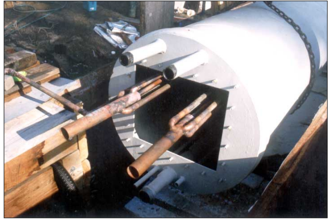
Left: Manoeuvring the 3000 litre storage cylinder into its final position, before boxing it in and insulating it. Right: One end of the 3000 litre storage cylinder, showing the access hole with the swimming pool water heat exchangers prior to final positioning.
