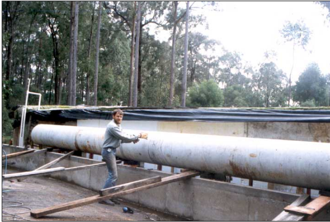
Left: Manoeuvring the 3000 litre storage cylinder into its final position, before boxing it in and insulating it. Right: One end of the 3000 litre storage cylinder, showing the access hole with the swimming pool water heat exchangers prior to final positioning.
