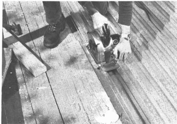
Cutting the Absorber Plate Along the Rib
