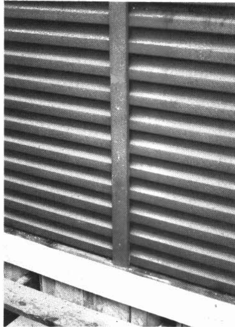
Fastening the Center Batten
