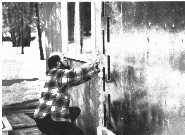
Caulking the EPDM End Closure Strip
