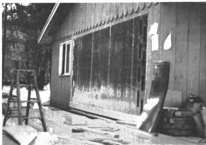
Thermo-ply Sheathing and Manifold Slots in Place
