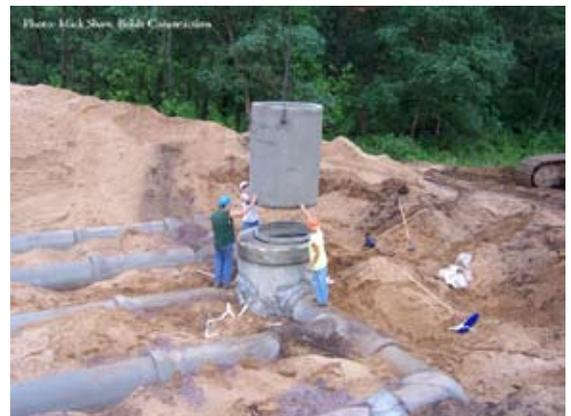
*Lowering the air intake tube into place. This piece will remain above-ground.*
