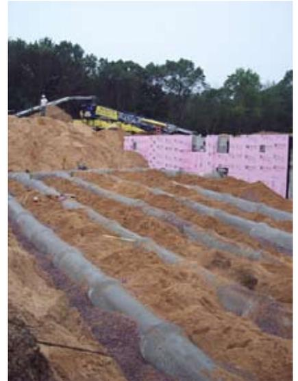
*The tubes connect to mechanical ventilation systems in the main building basement*
