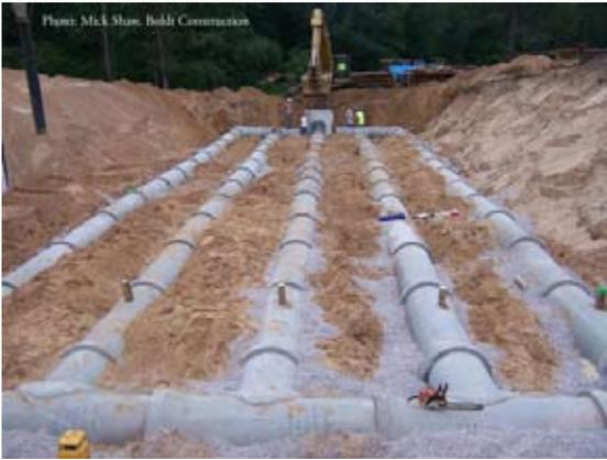
*Completed earth tube array*
