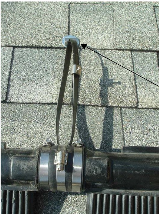
Figure 1: Mounting top header
