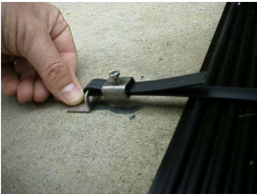
Figure 3: Strap, strap clamp, and strap bracket at end of a bank of panels
