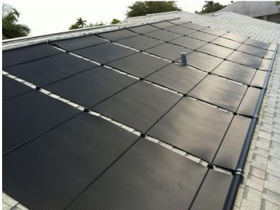
Now if you look at commercial pool collectors(mat style). There is a large header usually 1.5-2" and the riser(loops/pathway) are very tiny. Something like .25". Water goes rushing into the large header now a little bit goes through each tube and join back up on the other side. These little tubes use much less material, and thus is more efficient with material.
