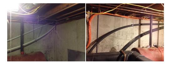
**Supply and Return Lines in Basement**: The picture on the left is before the lines were insulated and supported to the wall. The picture on the right the lines are both insulated and supported. One line feeds into the tank (not shown).
