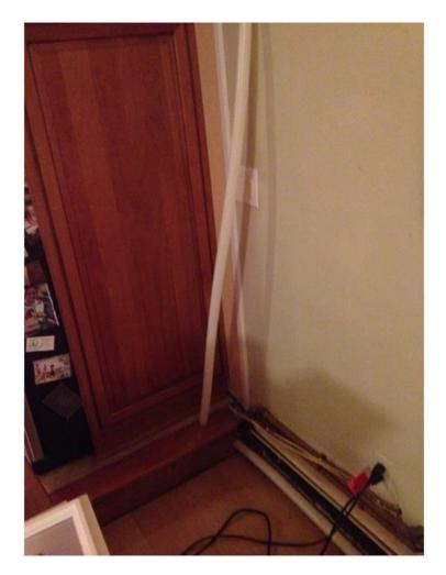
**Supply and Return Lines**: A chase will be built to cover the plumbing. Supply and return lines will also be insulated. The vertical line is the hot return coming from the crawl space. The lower line is the cold supply line feeding the bottom of the collector.
