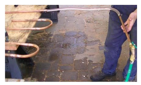
**Hooking the Hose to the Copper Ciricuit**: A straight piece of copper piping was soldered to a hose bib. Inexpensive C-Clamps were obtianed from the hardware store, with some plastic tubing to allow for easy on / off method for leak testing.
