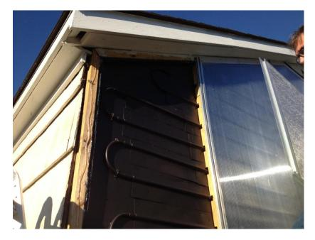
Adding the Last Piece of Twin Wall Polycarbonate: Note the heavy bead of silicon along the perimeter.
