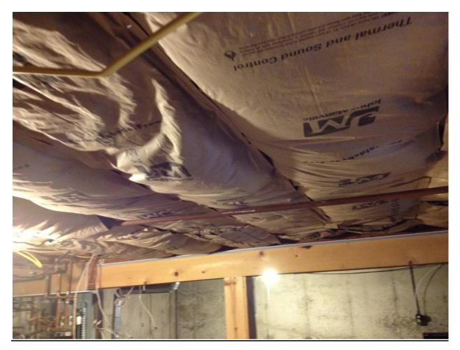
**Insulating Between Floor Joists**: Heat loss from the first floor of the home is minimized by adding batt insulation. This also insures the heat from the radiant floor heating system goes up into the first floor of the home instead of down into the basement.
