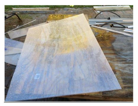
**Polycarbonate Cut on an Angle:** Saw dust and debris would get inside the twin walls, so we used a hose to clean out the polycarbonate before mounting. Moisture would dry out over time.
