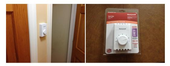
Thermostat Mounted: Use Drywall Anchors to mount thermostat to the wall
