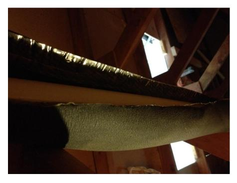
**Insulating the Pipe:** All piping to and from the collector should be insulated, especially the hot (return) line. Insulating was easy; just remove the adhesive tape and touch the tabs together.
