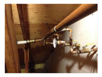
**<u>Copper to PEX Transition</u>**: All copper to PEX transitions were performed using shark bite Connectors.
