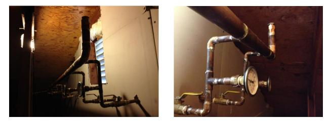
**Top Manifold:** Vacuum breaker shown, note vacuum breaker must be at the high point of the circuit.
