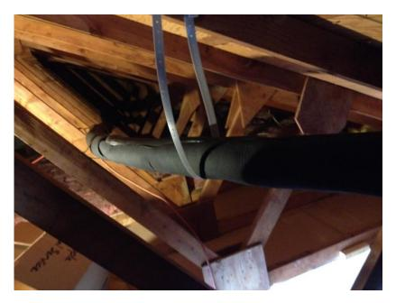
**<u>Return Line Through Crawl Space</u>**: Plastic pipe hangers were used to secure piping. Note that all piping was sloped at all times, especially since this is an unconditioned space.
