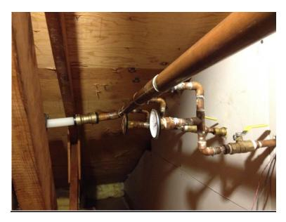
**Top Manifold:** Notice the sloping of the line, the temperature gages, shark bite connection and electric wires for both the temperature sensor and data logger.
