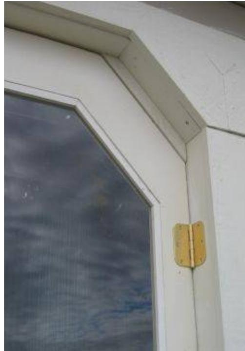
*Illustration 4* Note filler on frame to allow door to open fully
