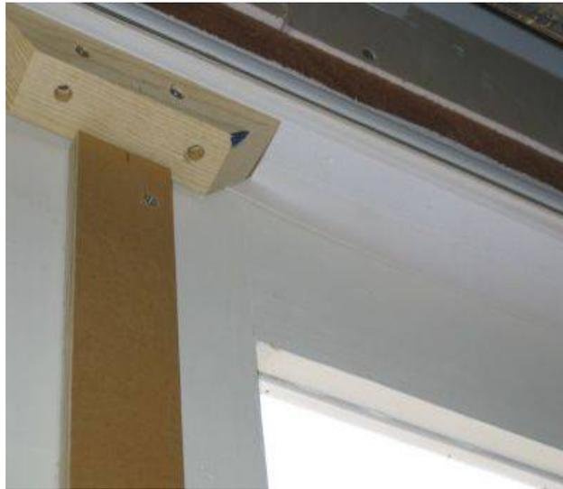
*Illustration 6* Detail of doors showing gap sealing strip and stop
