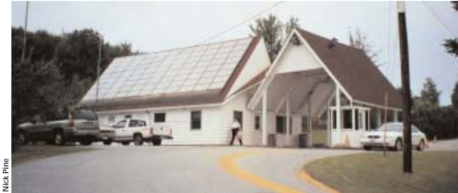
This 704 square feet of Harry Thomason's trickle collectors have been providing two-thirds of the Richford Customs House's heat since 1984.
