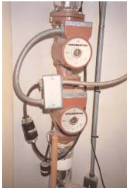
The solar system uses simple, reliable hardware, such as these two Grundfos pumps installed in series that move water from two 700 gallon tanks in an insulated rock bin up to the roof ridge line above the collector.
