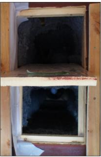
the fans turn on, the foamboard gets nearly perfectly horizontal (as shown in the picture) minimizing air flow resistance.
