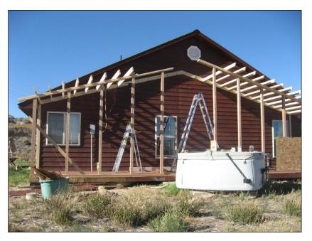
easy to score and cut. As shown in the picture the lower glazing area is 3'x3'. These dimensions handle the wind with no problems. The upper glazing area is 3'x6', and it wobbles too much in high wind. Someday I may add a brace, but it's nice to have the unobstructed view.
