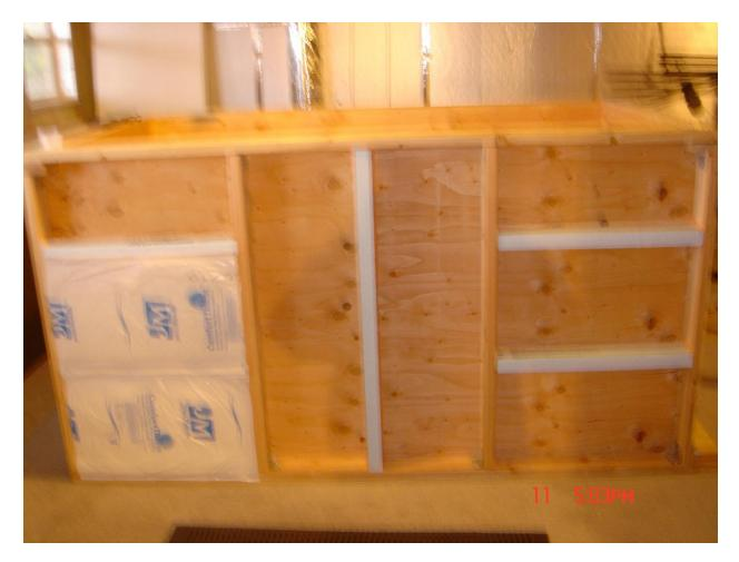
In addition to the 2" polyisocyanurate insulation on the inside of the tank, I added fiberglass batting between the 2x4 framing. As the spacing for the framing was not conducive to standard batting width, I created some structure from 2" polystyrene insulation. I held this in place with expanding foam. The plastic casing of the batting was attached to the foam with spray on adhesive.
