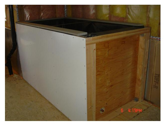
As a finishing touch I covered the walls with white water resistant wall board. On the lower corner of the end wall you can see the tank output which will go to the pump.
