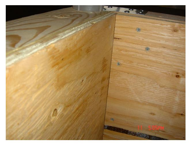
Inside corner of tank without extra corner piece that Gary and others have added. This piece is not needed because of the extended side walls. This square corner makes fitting interior 2" insulation easier.
