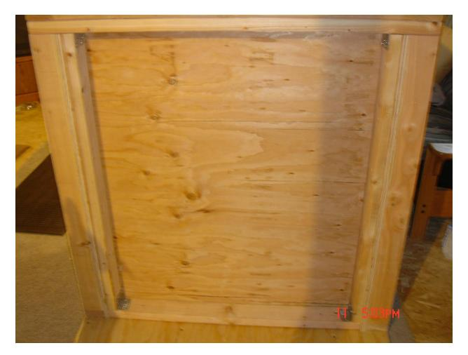
I extended the long sides of the tank walls past the end wall and I believe this provides much more support. Note how the vertical 2x4's clamp the extended plywood and the end 2x4's can be screwed into by both the long side and the short side.
