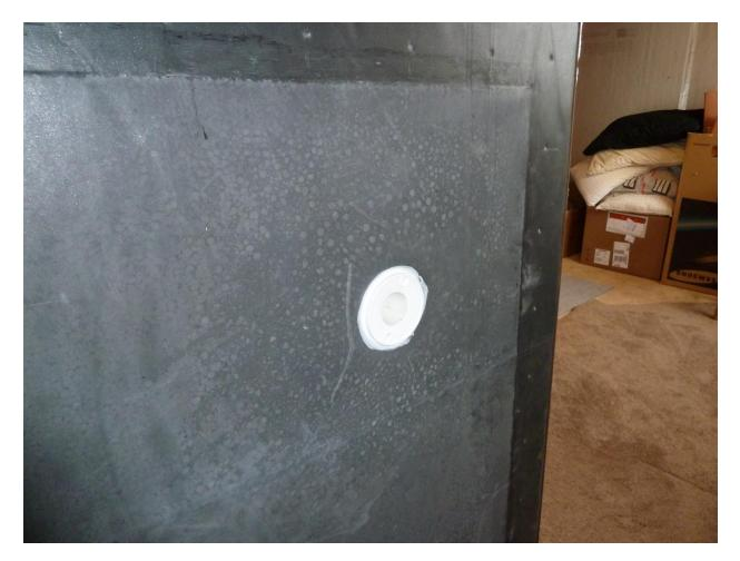
The inside connection of the access hole is a floor drain flange siliconed to the EPDM material.
