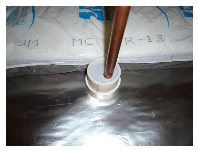
The return access hole though the lid is limited in size with a modified pipe cap.
