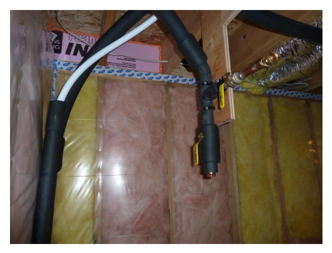
The right side connection with the ball valves is the return from the solar panels. I used PEX-AL-PEX for the connections between the solar panels on the roof and the solar tank in the basement. As the lid was off during this picture the piece of pipe that extends into the tank has been removed.
