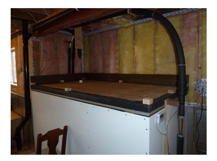
The lid is a layer of EPDM wrapped around 2" of polyisocyanurate and stapled (with stainless steel staples) to a sheet of 1/2" plywood. The small wooden blocks are for attaching the lid walls. On top of the plywood I put another sheet of 2" polyisocyanurate followed by a layer of r13 fiberglass bats (r39 total).
