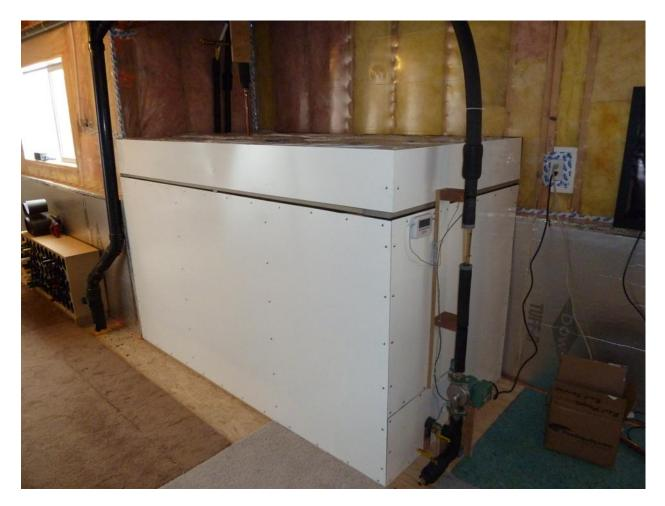
The tank design was based on your plywood, EPDM liner design.
