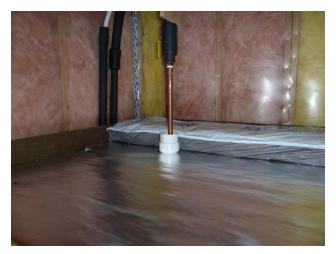
This shows the lid and the solar panel return line. I decided to run the pipe straight through the lid and when I need to remove the lid I unscrew the short length of copper pipe. Having a straight shot like this improves the ability to break the syphon.
