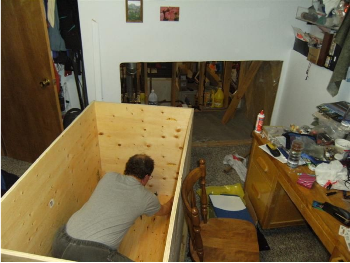
Tank construction. Note hole in drywall where tank will go through.
