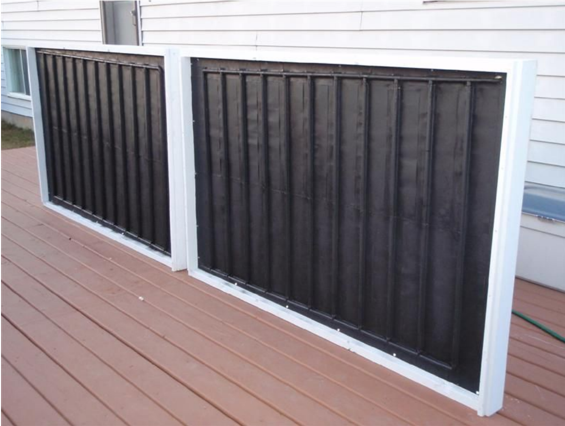
Collectors before glazing went on
