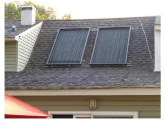
Collectors in rails on roof before connecting everything together and closing them up. They sit about 2-3 inches off the roof. Notice the return line inside the left collector. I figured it made more sense to keep the line inside the collectors to maybe get some additional heat. So it passes through the right collector as well before dropping inside the house and down to the tank.
