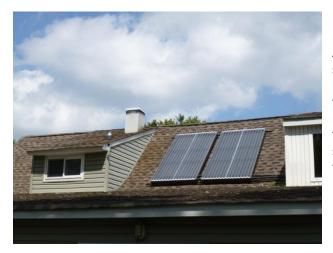
Finally, everything is connected and sealed up on the roof. I'm very happy with the final look. After nearly two weeks running my Kill A Watt meter is saying it is costing \$1.92 a month to run everything. I'm not thrilled with that but unfortunately being about 18 feet from the pump to the top of the collector, I have to run the pump on the highest speed on startup. I'd like to figure out a way to use a second pump once the system starts and shut off the main one to cut down that monthly cost.
