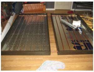
Dry fitting to make sure everything will still line up when I attempt to connect the two collectors together on the roof. I connected the panels together with ¾ in Sharkbite connections so I could easily take everything apart if necessary. All of the exterior plumbing is wrapped in that rubberized insulation they sell at Home Depot.
