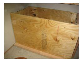
The tank is roughly 60Lx36Wx39H. I used 2 inch polyiso insulation on the inside walls and bottom plus another 2 inches of polyiso on the floor below the tank.
