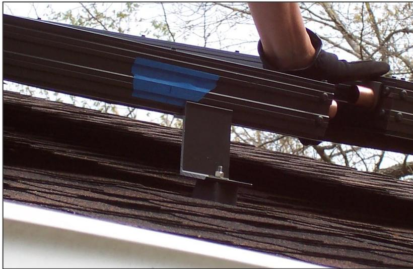
If I had it to do all over again, I would still use the Quick Mount PVs, but I would set them in a 3 x 3 grid, run U Channel across the QMPVs in 3 horizontal runs, and then mount the collectors to the U Channel "rails" using the AE-RM brackets. In hindsight, this would have made setting the proper drainback pitch as well as aligning the couplings much easier – though with careful planning, measuring and execution, the way we did it was not that difficult.
