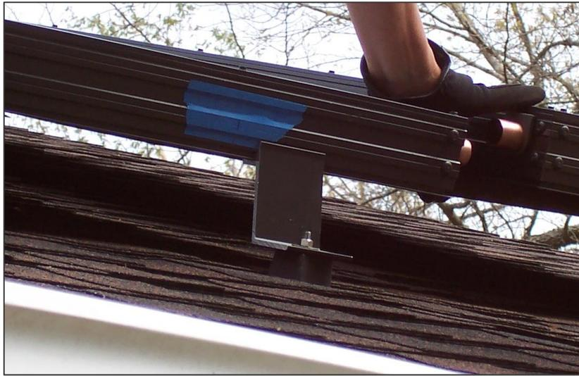
Having selected AET brand commercial collectors for our system, the next step was to figure out how to mount them. Not wanting ground mounted collectors due to the visual impact, we decided to place them on the roof of the garage with a perpendicular azimuth of 139 degrees (SE) with a pitch of 43 degrees. Our latitude is 36.83 degrees, so after studying the de-rates due to azimuth and elevation, we decided that fixed mount on the roof plane would be "close enough".
