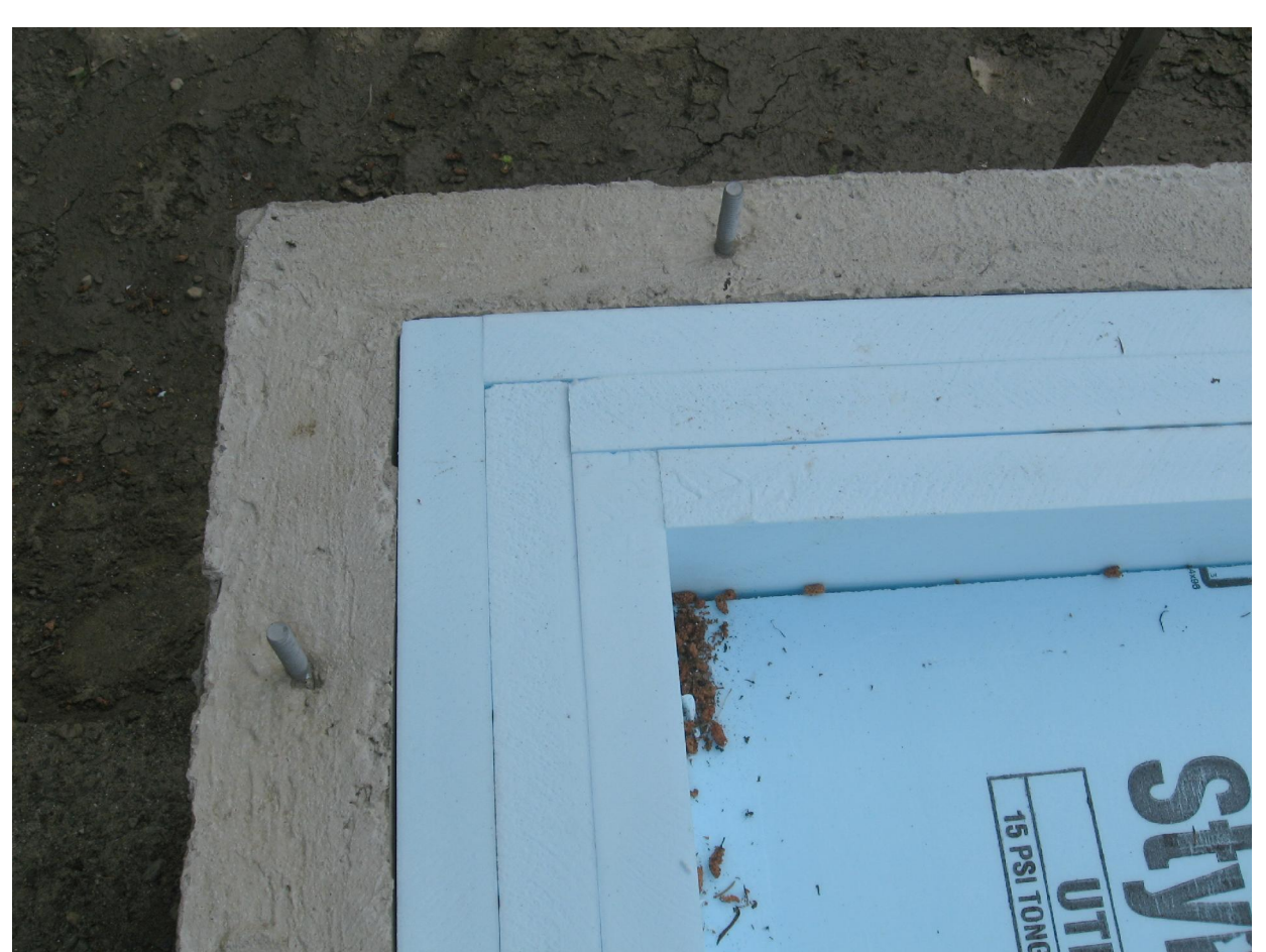
SLAB IS FULLY INSULATED
