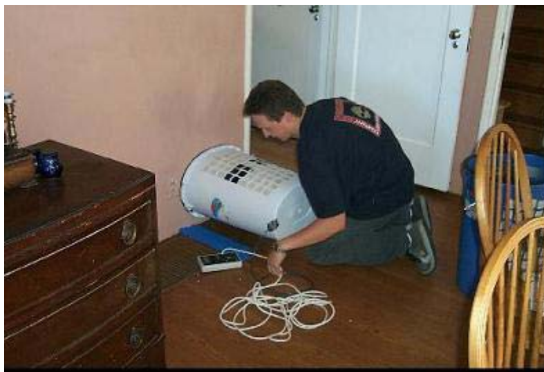
Figure 3. Residential supply airflow measurement
