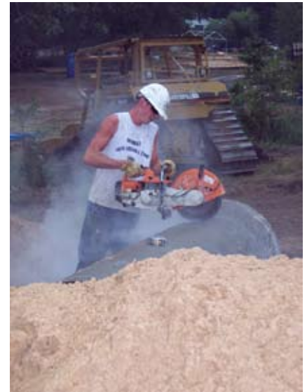
Cutting tube to length
