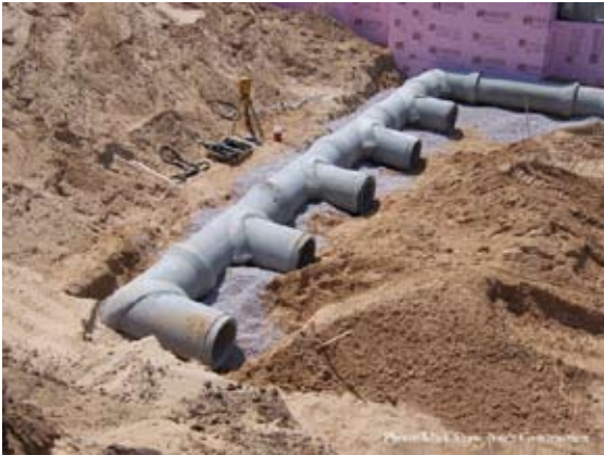
Laying the earth tubes begins
