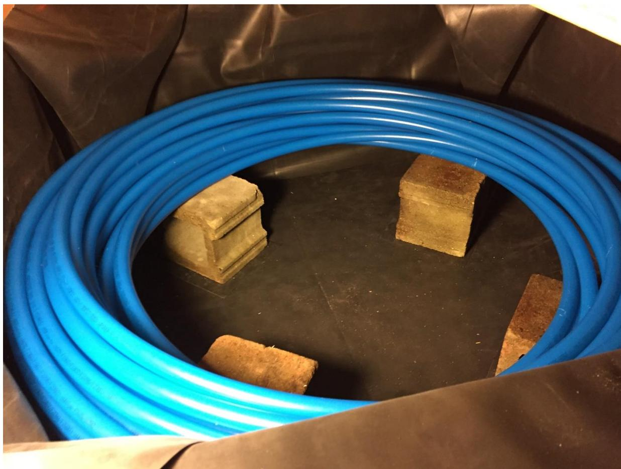
Coil of PEX tubing inside tank, 300 feet, one-inch nominal.
