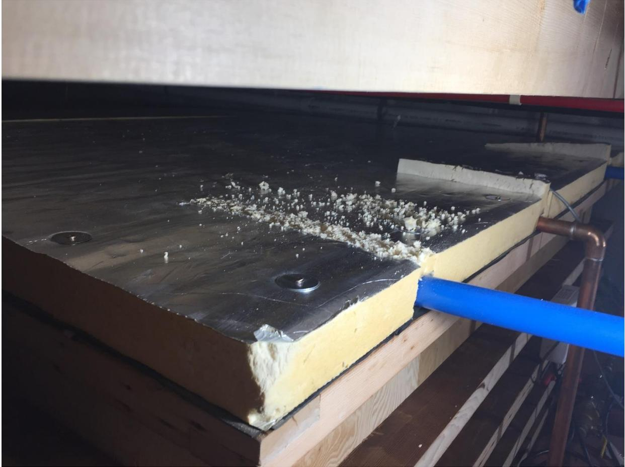
First layer of foam is screwed in place, and cut to fit around pipes.
