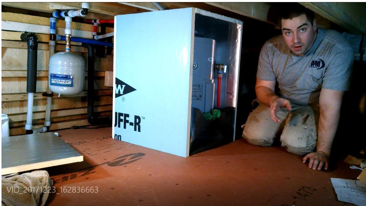
Electric booster tank inside an insulation box.
