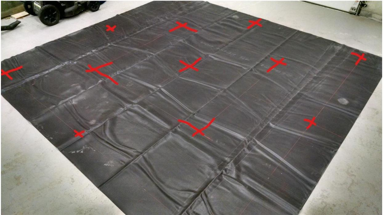
Chalk lines snapped out on EPDM prior to installation.
