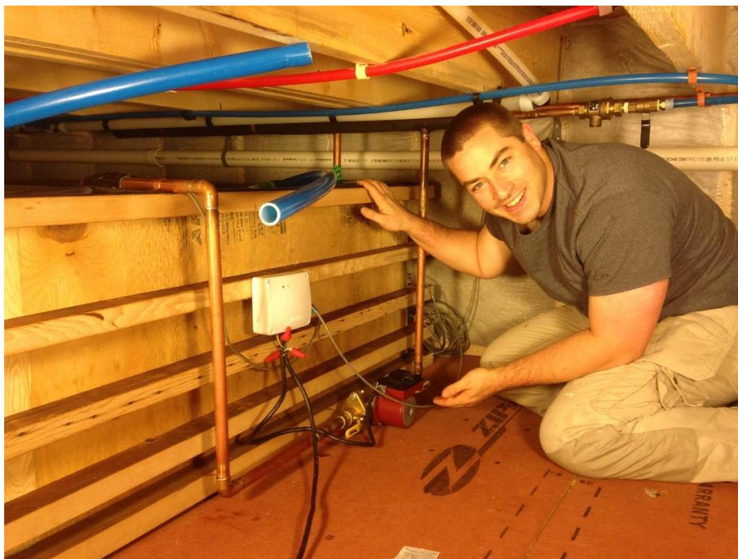
The pump is red, near the floor, and the controller is the white box mounted on side of tank.
