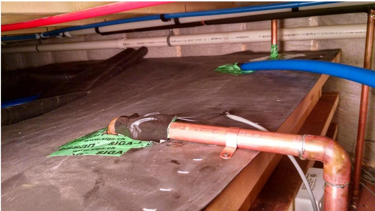
Pipes entering the tank through the lid with gasketed seals. Note the temperature sensor is taped to the copper pipe.
