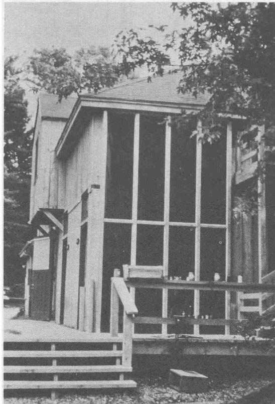
**Photo 2-1:** This 8-by-14-foot TAP was retrofitted onto the Hitchcock Nature Center in Amherst, Massachusetts. It heats the second-floor office space and uses an open stairwell as the cool-air return. This collector experiences some morning shading, which indicates that a little tree trimming is in order at this site.
