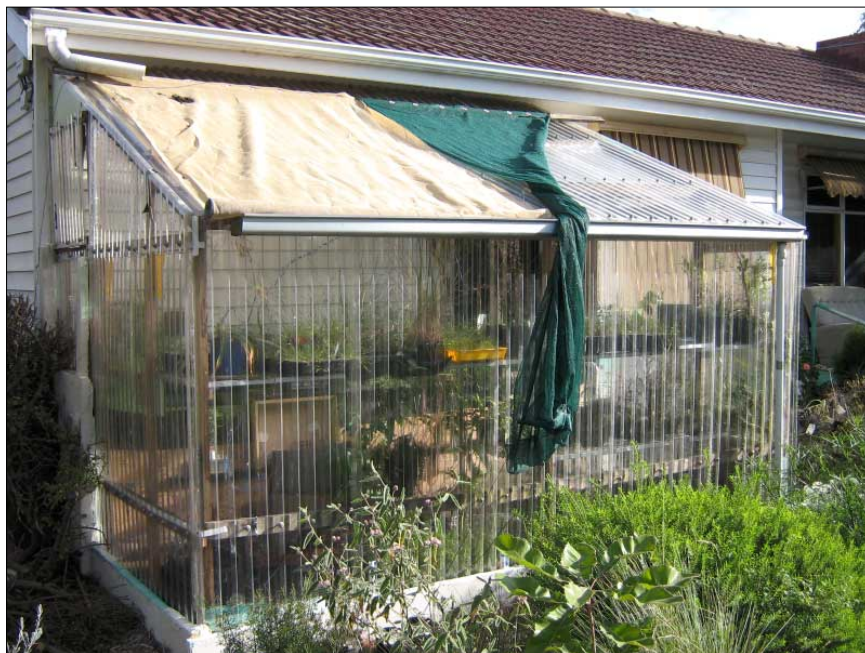
This greenhouse collects the heat for the storage system.
