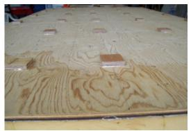
1/4 inch ply was glued and screwed. The stressed skin panel via the strips was glued and screwed to the 1/2 inch ply frame making it strong and rigid. This spruce also provided the perimeter seat on which the polycarbonate sheet sat (see section drawing).
