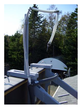
The air trap is just a tee mounted at the highest point of the plumbing with a straight vertical pipe and two 90 degree elbows. Any air in the system bubbles up into the straight pipe and stops circulating back to the pump.
