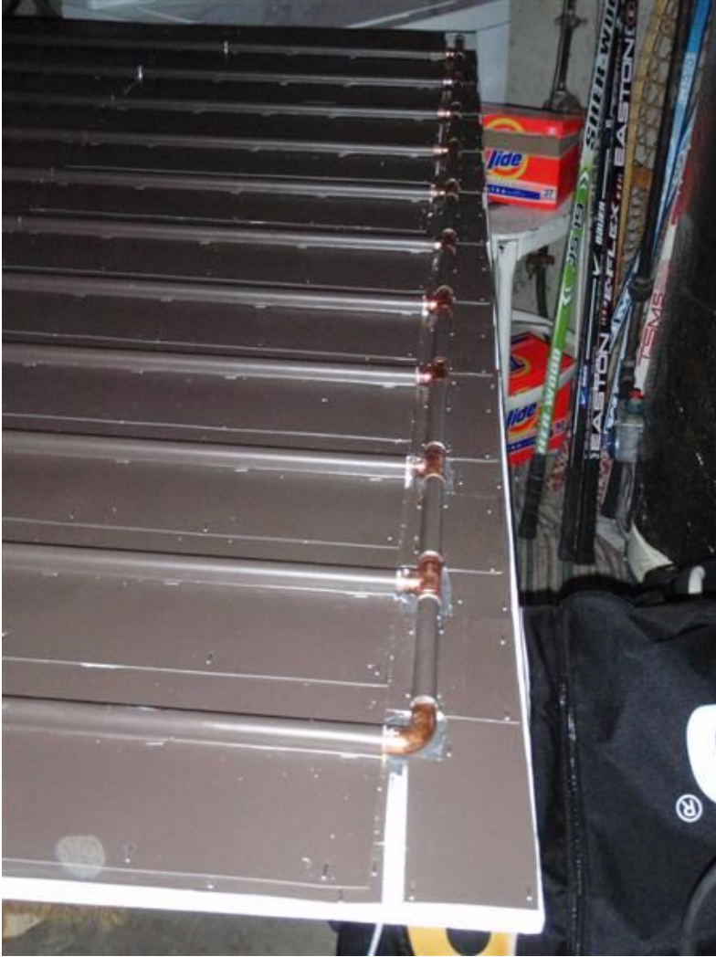
Top layer, showing overlapping flashing and coverage out to edges
