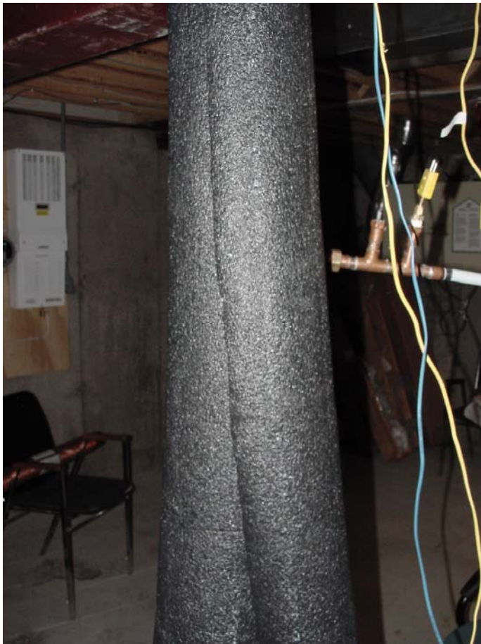
Figure 2: Insulated DWHR
