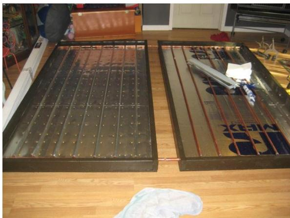
Dry fitting to make sure everything will still line up when I attempt to connect the two collectors together on the roof. I connected the panels together with  $\frac{3}{4}$  in Sharkbite connections so I could easily take everything apart if necessary. All of the exterior plumbing is wrapped in that rubberized insulation they sell at Home Depot.
