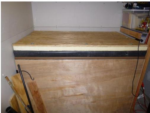
Lid installed and controller/pump hooked up to Kill A Watt meter so I can see how much energy I'm using to run the system.
