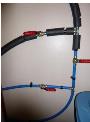
3 ball valves which allow me to bypass the entire system by turning off the two horizontal ones and turning on the vertical one.
