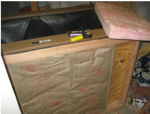
I added additional R-13 insulation to the outside to get a higher R value and hopefully lessen standby loss.
