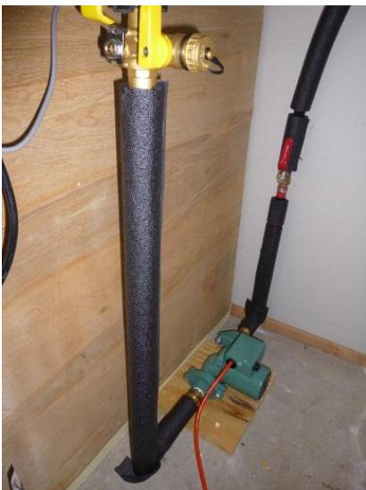
Here is the U-Tube arrangement. The top yellow handle allows me to hook my hose up to the line to add water and prime the pump. Just to the left you can see the ball valve handle. This was a nice single piece that served both functions. I got it from PexUniverse.com for \$11.95. It's called
