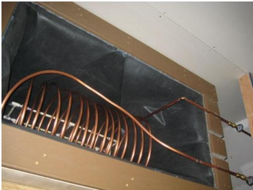
I also added two temperature gauges (one just before the cold water enters the tank, the other right after it exits). These are  $\frac{1}{2}$  in Sharkbite Temperature gauges which cost about \$30 bucks each (PexUniverse and Home Depot carry them) but it makes it easy to see incoming and outgoing water temperature when running hot water. At this point I ran some tests and did not see any noticeable difference on water pressure when drawing hot water through this additional length of copper.
