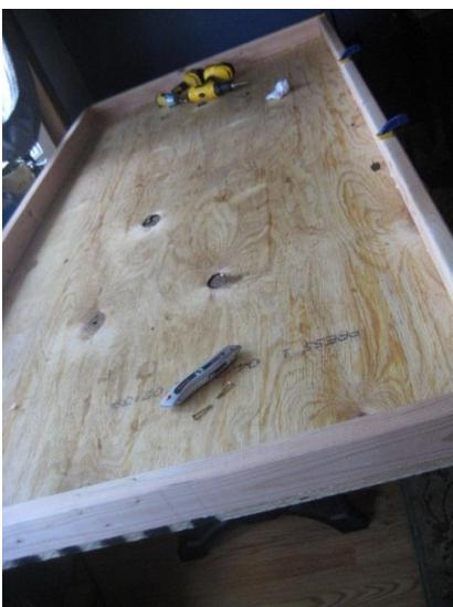
Building the frame for the collector. It's made of 2x4s and  $\frac{3}{4}$  in plywood and painted with a few coats of exterior paint.
