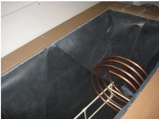
I decided to go with copper since I had read in a few places online it was 4 to 5 times better at transferring heat than PEX. Whether that is accurate or not I don't know but I went with a total of 80 feet of  $\frac{1}{2}$  inch Type L soft copper. I went with a wider diameter figuring that the copper was spread through the tank more so on longer draws it would pull heat from a larger volume of water more evenly. Not sure if it matters but the heat exchanger is working very well regardless.
