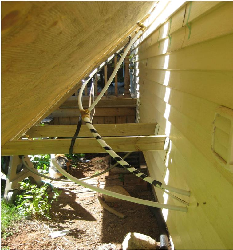
*Illustration 1: Return line is visible. Electric tape holds the sensor wires against the lines*
