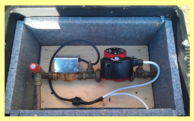
The pump is positioned on the return with the PRV after the motorised valve.
