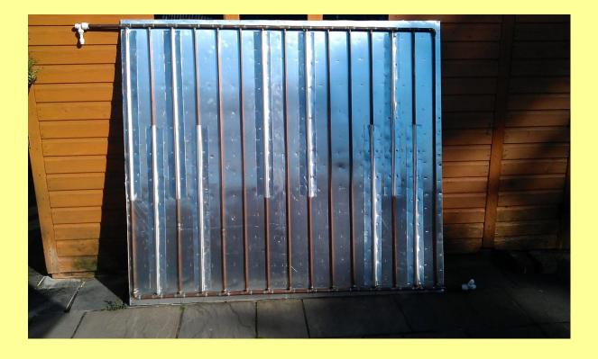
Once fully covered I sprayed the manifold with black baroque paint and made the framework for the manifold to fit in with 96mm x 20mm soft wood. This was lined with 25mm polystyrene insulation board
