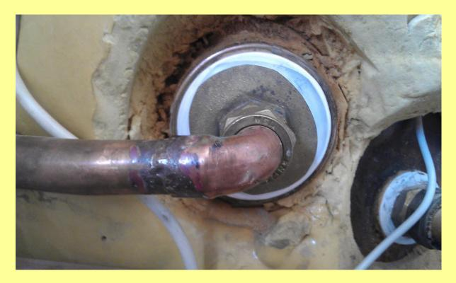
I took out my immersion heater to incorporate a connection at the bottom of the cylinder. An immersion heater in a thermal store is used as a back- up heat source if the boiler breaks down. There about as good as a chocolate tea-pot on this cylinder. I fitted isolation values on the flow and return to the solar panel so it can easily be drained down in winter time along with a flow meter so I can set up the correct flow speed through the solar panel.
