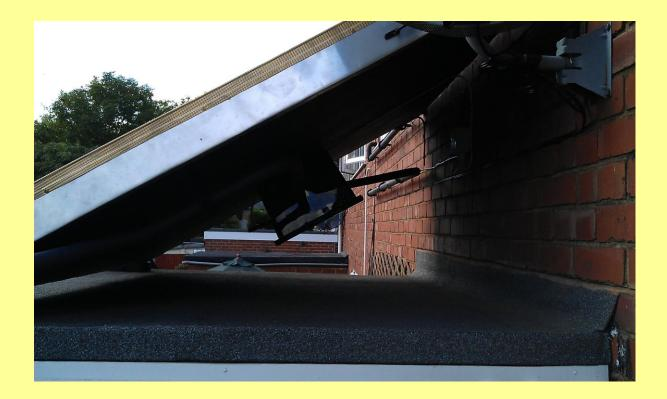
The panel was piped to the cylinder in 22mm copper using soft solder and compression fittings, externally, with brazed and compression internally.
