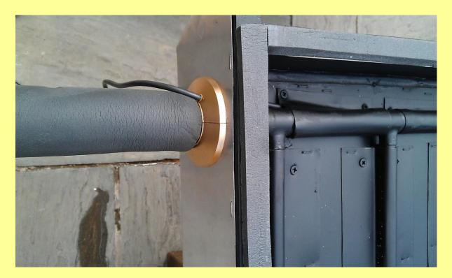
The external pipe-work was insulated with 12mm thick armaflex to stop heat loss.
